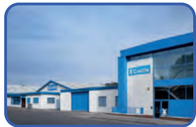
Castle Precision Engineering £35m contracts secured
